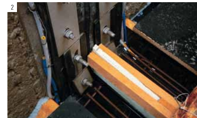
1+2 Posing and fixing of joint tape prepared in-situ and completion of reinforcement 3 Adjusting and flanging of special construction at the transition floor – wall
