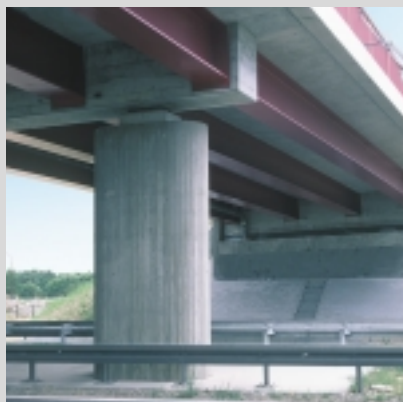
Completed double-span bridge over the motorway
